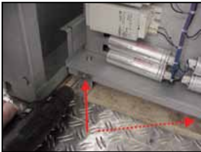
22. Remove the shipping brackets from the service tray. (Figure 16)
