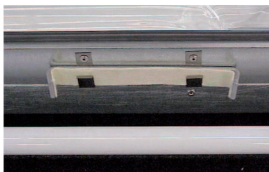
Illustr. 5-5 Suspension of the base pane
