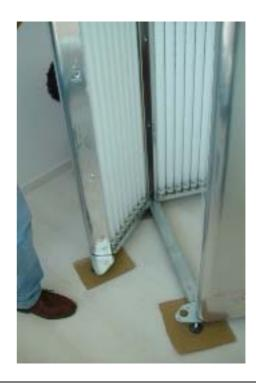
Panel 3 has no brackets on the bottom, it has to be inserted between panel 2 and 4. Carefully place the screws on the bottom of the panels through the access holes in the mounting plate. Secure the panel in its place using the M6 nuts from the bottom.
